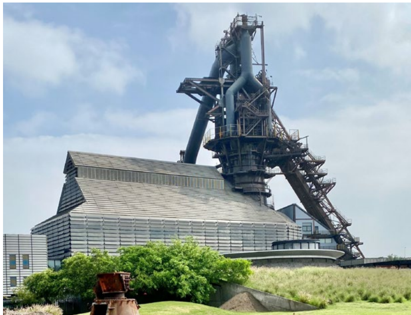
Museo del Acero Horno 3', the blast furnace at the heart of Fundidora Park in Monterrey, Mexico, which hosted the 10th Latin American Colloquium on industrial heritage in October 2023 See page 3 . Photo: Miles Oglethorpe
