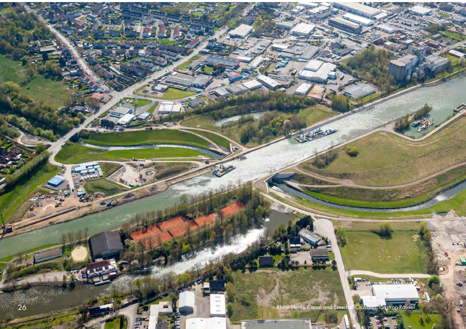
Wastewater Treatment Plant Bernemündung, Bottrop-Ebel
